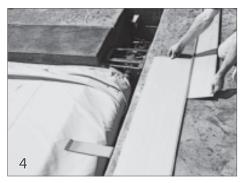
Assembling the Aluminum Lid Assemble the lid by sliding the hinge (16/17) onto the main section of lid (15).
