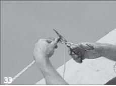
While pulling both ropes tight, use a lighter or torch to burn the rope in the location it will be cut. This will help them not fray after they have been cut. Cut the ropes so they are at least 8 ft long. Use the lighter to burn the cut ends of the rope if needed.
