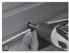
Install rope loops (25) on the rope along the back of the cover box. Secure the loops to the cover box using appropriate screws and anchors, depending on the type of cover box that is used.
