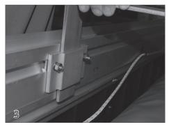
Slide the standard lid bracket into the drop in anchor plate.
