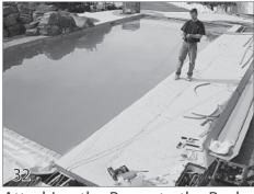
Attaching the Ropes to the Reels The cover must be open when cutting and attaching the ropes. Pull the cover back until the sliders are against the guides. Pull the ropes tight as they come off the pulleys on the mechanism to eliminate the slack in the rope.
