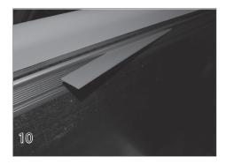
Insert and tap the locking strip into place underneath the track along the entire length of the track. Make sure a locking strip is placed at all track spices. Do this along both sides of the pool. The shim needs to end at the inside edge of the cover box.
