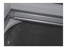
When encapsulation retainer is being used, the track is normally installed during the cover installation. With the track installed, make sure it is flush with the end wall at the shallow end.
