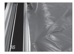
Distribute the slack of the cover evenly between each screw across the length of the tube. Secure the cover to the roll-up tube using #10 x 1/2" SS tek screws (36) every 2-3 feet.
