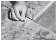
Insert plastic anchors (26) into the holes and tap with a hammer so they are flush with the deck. Fasten the lid to the deck with #12 pan head screws (40).
