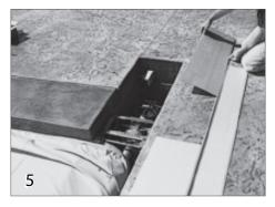
Slide the motor (18) and non-motor (19) ends onto the hinge.
