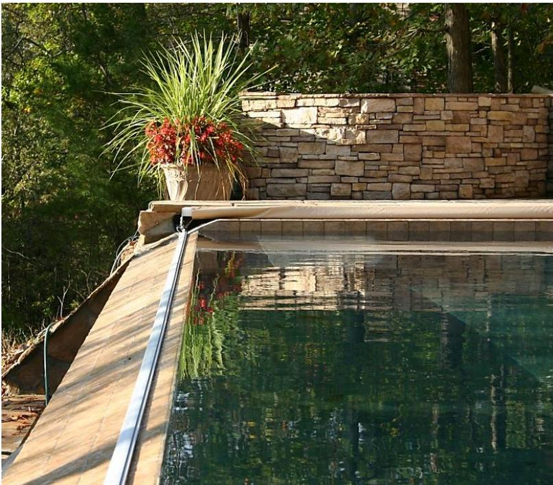
Note spacer under the track. Turn so that corner is pointing away from track. This allows water to flow around and under the track.
