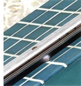
Bond Beam is slanted same as side bond beam. Slant area is 1/2" to 1" higher than side of bond beam.
