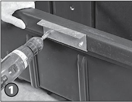
Install the "z" mounting brackets (3, M9345) on the lip of the polymer housing every 24-26 inches. Fasten each section in place with 1" tek screws (1, A1700).
