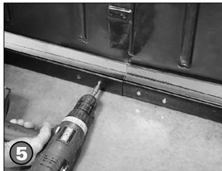
5 Fasten both splices into place with two 1" tek screws (9, A1701) per splice. Repeat this process to complete the assembly of the polymer housing.
