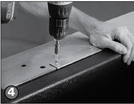
Fasten the "z" channel bracket (3, M9345) to the top of the pool wall using 1" tek screws.
