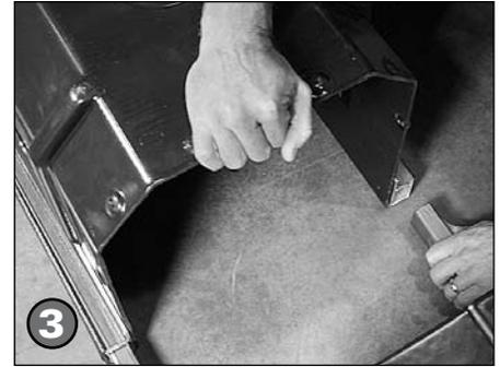
3 Slide polymer housing sections together and join ends tightly.
