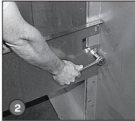
Place polymer housing support brackets (4, M9787) 14-1/4 inches below top of pool wall (See Side View, bottom of page), cutting braces as necessary. Bolt into place using wall joining hardware supplied by the pool wall manufacturer
