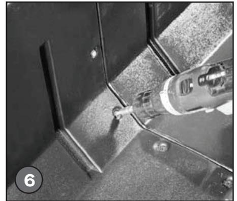
Fasten the sections together from the inside of the housing to the outside with six 1" tek screws. Repeat this process to assemble the full length of the polymer housing.
