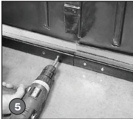
Fasten both splices into place with two 1" tek screws (9, A1701) per splice. Repeat this process to complete the assembly of the polymer housing.
