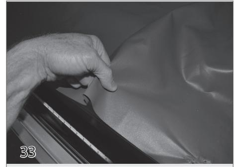
Find the center of the slack and pin directly to the tube (DO NOT FOLD THE SLACK). Repeat this step several times along the tube.
