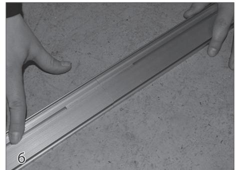
Continue tapping the end of the track until the two sections of track are tight together so there is no gap between the lengths of track.
