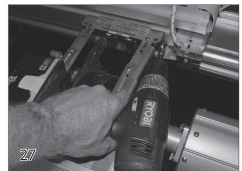
Position the fabric on the leading edge so it is in line with the edge of the rope C-channel. Pin the rope hem to the leading edge by placing a #10 x 5/8" pinning screw (41) in the drilled hole and through the rope hem.
