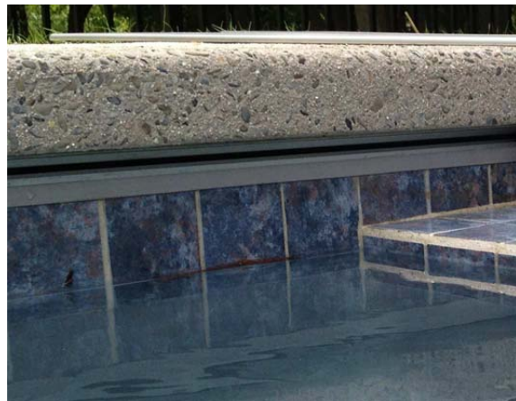
Exposed Aggregate Concrete
