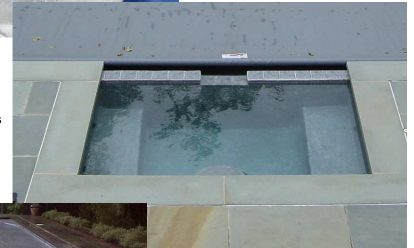
Open Spillway Used only on end wall spas
