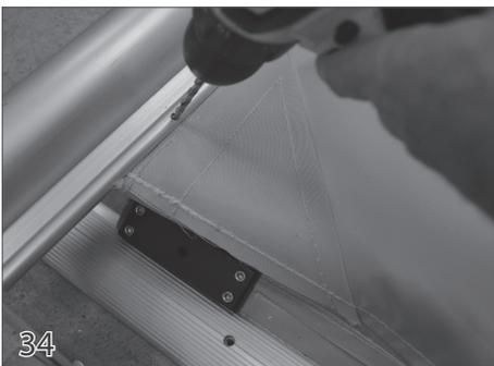
Center the cover on the leading edge. Distribute the slack towards the center of the leading edge. Make sure the corner gore is upright and does not contact the pool deck. Use caution when drilling near the cover.
