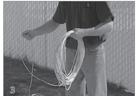
Uncoil the ropes to remove twists and kinks. Run the ropes through the tracks. There are two methods that can be used.
