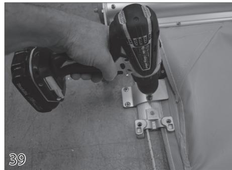
Reinstall the guide on the end of the track. Secure the Positive Stop Plate to the top track using the 1/2" x 3/4" screws (32) provided. Drill and anchor through the other holes of the positive stop plate into the pool deck. Secure the stop plate to the deck using the screws (29) and anchors (16) provided.
