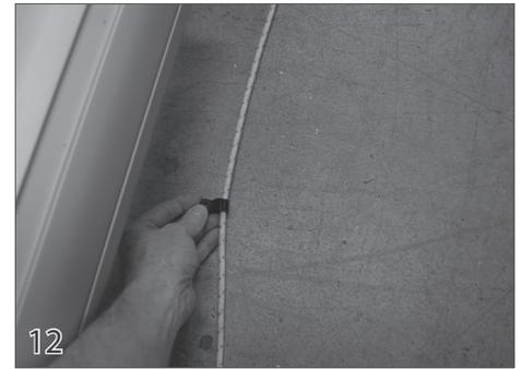
Run the rope from the non-motor end along the pool deck behind the mechanism. The rope should run through the rope loops (15) to keep it from getting caught in the cover. Space the rope loops evenly behind the mechanism.
