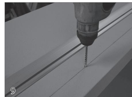
Drill 1/4 inch x 1.5 inch deep holes every two feet along the chalked line on both sides of the pool.
