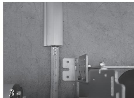
Cut the length of the track on each side of the pool so it will be about 2 inches from the mounting foot at the mechanism end, and 18 inches past the end of the pool at the shallow end.
