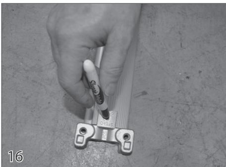
Using the guide (12) as a template, position it on the end of the track. Mark the center of the mounting hole.
