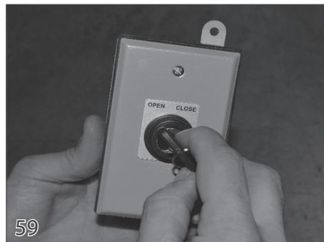
59 Run the key switch in the open position to roll the cover up on the roll-up tube. Check the cover to be sure it rolls up evenly. Run the cover 6-10 times to make sure it opens and closes evenly. The cover fabric installation is now complete.
