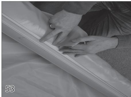
Distribute the slack of the cover evenly between each screw across the length of the tube. Secure the cover to the roll-up tube using #10 x 1/2" SS tek screws (23) every 2-3 feet.
