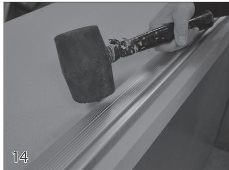
Using a rubber mallet, strike the center of the track to secure it to the snap-locks. Be sure the track is flush with the pool deck.
