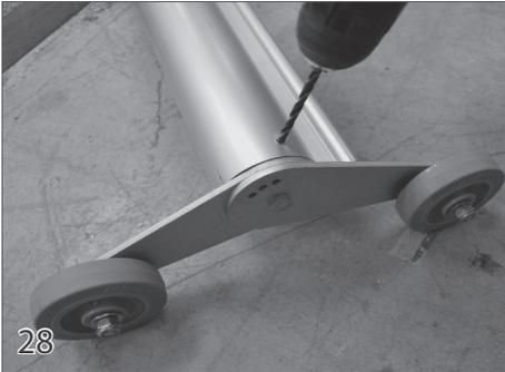
Drill a minimum of three pilot holes evenly spaced around the leading edge and into the white dowel.
