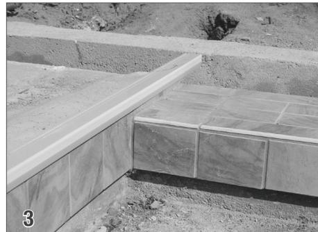
**3 Place the Encapsulation** If encapsulation is installed before the tile, overhang the encapsulation 1/2" into the pool aligned with the string line. If the tile has already been installed, place the encapsulation flush with the tile.
