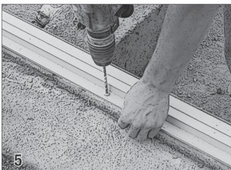
**5 Drill Holes in the Wall** Drill through the back flange of the encapsulation 2 1/2" deep. These holes should be placed every 24 - 30 inches.
