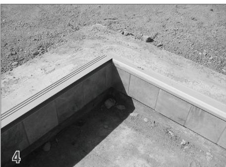
**4 Miter the Corners** Begin at the end of the pool opposite the cover mechanism. Miter cut a 45 degree angle on the ends of two lengths of encapsulation. Place them together on the corner to form a 90 degree corner. Make the same cuts for the other corner of the pool. Continue placing lengths of encapsulation around the rest of the pool. Cut the encapsulation so it will extend 1 inch into the cover housing.
