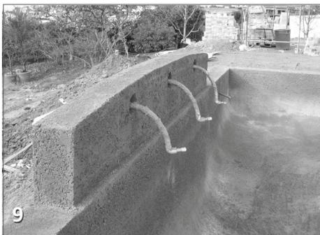
**9 Optional Raised Wall** Pools with raised walls can also be formed with a three inch ledge. The encapsulation is anchored to the ledge, allowing stone to be set in place on top of the encapsulation. It is important that the track and spacer be inserted into the encapsulation to prevent it from collapsing.
