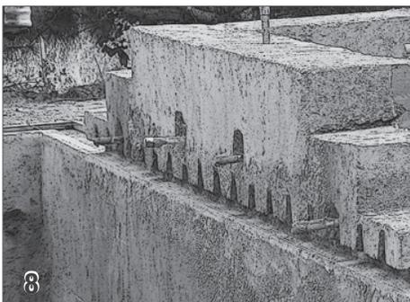
**8 Optional Raised Wall with Pocket Holes** Pools with a raised wall need a cavity large enough to accept the encapsulation (3"x 2") and should have pocket holes formed to allow it to the encapsulation to be screwed into place.
