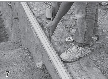
**7 Fasten Encapsulation in Place** Place the encapsulation back over the holes and anchors. Secure the encapsulation to the pool walls by inserting a hex head screw and tightening with a drill. Tip: Install track and spacer in the encapsulation to help the encapsulation and corners line up straight while it is being secured to the pool wall.
