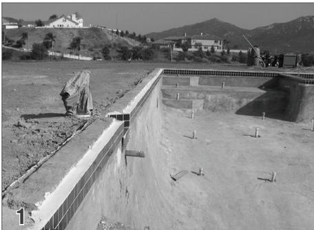
**1 Mortar A Level Mounting Bed** Mortar the top of the gunite walls so they have a 3" min flat, straight and level surface for the encapsulation to be mounted to.
