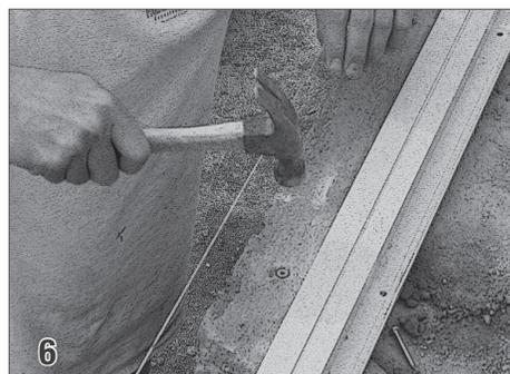
**6 Tap in Anchors** Move the encapsulation back a few inches to expose holes. Insert plastic anchors into each hole.
