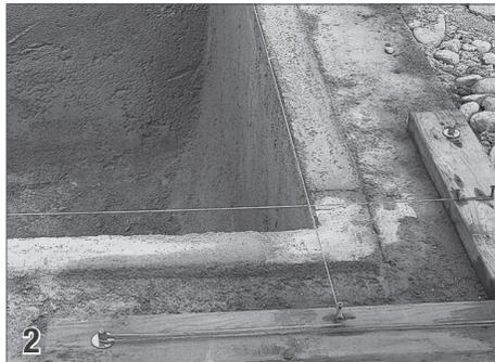
**2 Square the Pool** It is recommended that the encapsulation be secured to the pool wall after the tile has been installed. If the encapsulation will be installed before tile, run string lines around the pool to create a perfectly rectangular pool.
