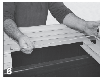
6 Using the piece of riser that is 40 inches long and notched at each end (M9354), cut the riser to fit on the front side of the housing for the motor and non-motor ends. The cover guide will pass through the notches in the riser.
