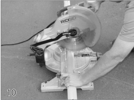
Cut the track at the mechanism end to the proper length using a miter saw. It is important to have square cuts on the track. Note: Always wear safety goggles when using powered equipment.
