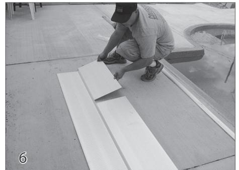
Slide the motor and non-motor lid ends onto the hinge.
