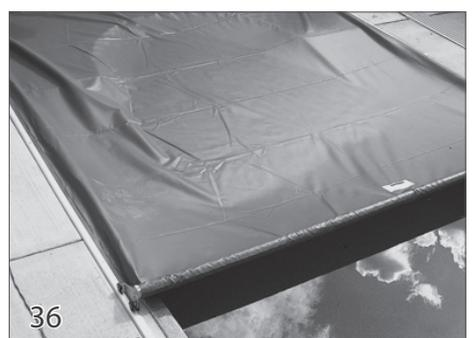
Run the key switch in the uncover position to roll the cover up on the roll-up tube. Check the cover to be sure it rolls up evenly. Run the cover 6-10 times to make sure it opens and closes evenly. The cover fabric installation is now complete.
