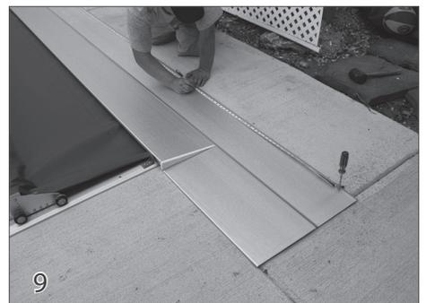
Measure across the hinge to evenly space the screws. Continue drilling and anchoring the hinge in this manner until the entire lid is attached to the deck. If any part of the lid is sticking up, it must be screwed down to the deck. The safety pool cover installation is now complete. Now instruct the home owner using the home owners guide and the checklist on the next page.
