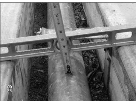
With the mechanism and tube assembled and set in place in the housing, check the roll-up tube for level. This is crucial for proper operation of the cover. Position a level across the housing. Measure from the roll-up tube to the bottom of the level on both the motor end and non-motor end of the mechanism. Adjust height of the non-motor end feet if needed to level the roll-up tube.
