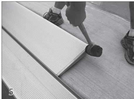
Slide the plastic wedges (15) onto the main lid on either side. Tap into place with a rubber mallet.
