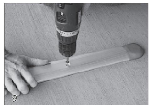
Complete the fastening of all track screws flush to the top of the track and fasten the pulley screw on both sides of the pool. Clean concrete dust from tracks and pulley endcap. Make sure ALL screws are flush with tracks.
