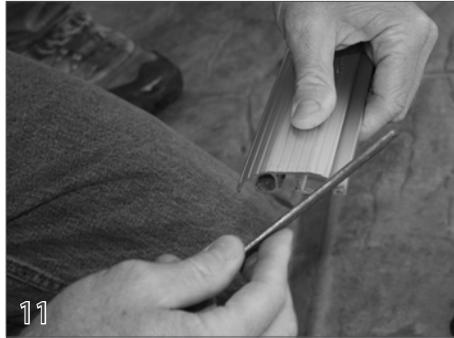
File the track ends on both sides of the pool making sure to round all edges and remove all burrs. This step is extremely important. The cover can be damaged very easily by metal burrs and this damage is not covered by the warranty.
