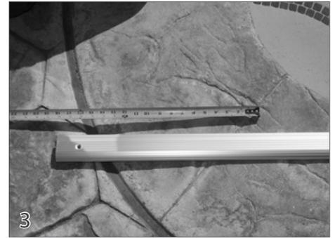
Extend the tracks at least 18" past waterline. Center the pool shape between the pool tracks where possible. Measure and mark the track space and track length on the deck.
