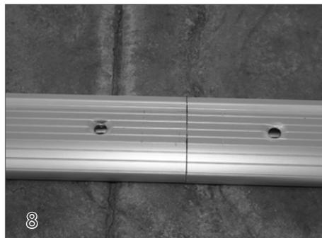
The two sections of track should be tight together.
