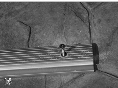
Place the track back over the holes in the deck. Fasten the track screws (34) halfway through the tracks into the plastic anchors. The screws will be fastened completely later in the installation.
