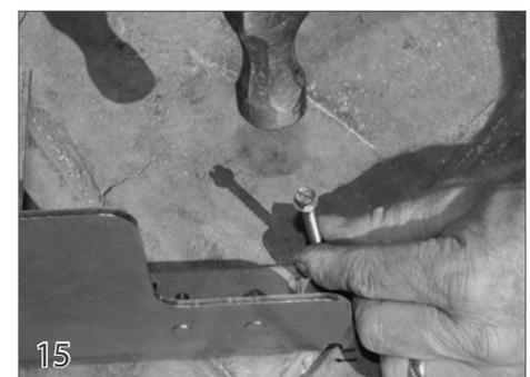
15 Use the 1-1/2" hex head screws (26) and anchors (25) provided to secure the motor end and non-motor end to the deck.
