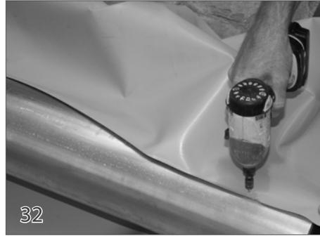
The first two screws need to be 3" from the end of the tube. Distribute the slack of the cover evenly across the length of the tube. Secure the cover to the roll-up tube using tek screws every 2-3 ft. When attaching the cover to the tube, do not use folds or pleats. Operate the cover 6-10 times to make sure it is opening and closing squarely.
