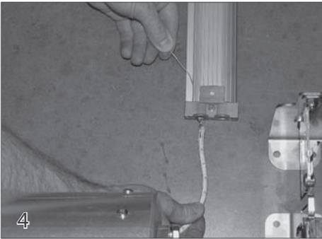
Feed the rope into the water side channel of the track with the wire extending out the side of the track. Use the wire to pull the rope down the length of the track towards the end of the pool.
