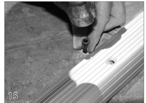
Move the tracks to the side to expose the holes in the deck. Clean the dust from each hole and tap plastic anchors (41) into each one.
