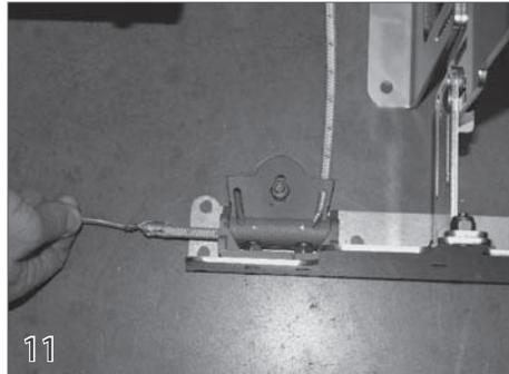
On the non-motor end, feed the wire that is attached to the rope around the pulley and out the back channel of the pulley assembly. Pull this rope to the motor end pulley assembly.
