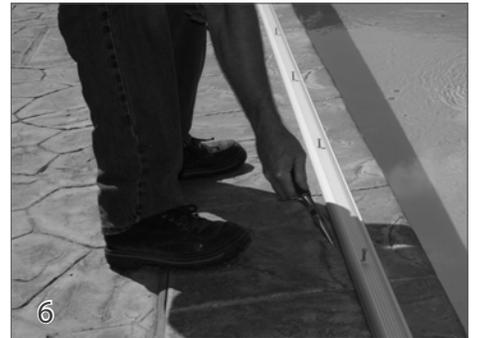
Feed the rope into the back channel then pull the rope down the back side of the track toward the cover housing.
