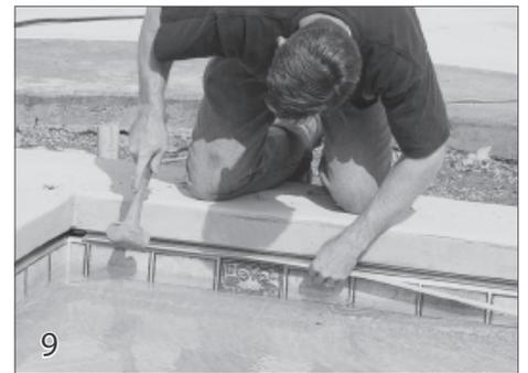
Install the spacer underneath the track to lock the track into the encapsulation.
