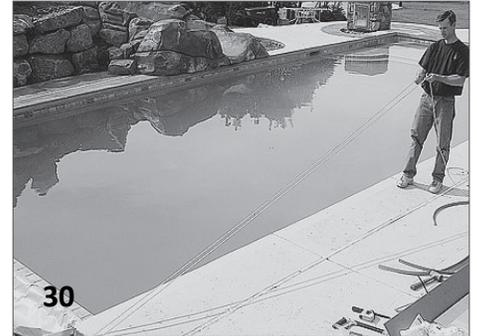
Leaving an extra 6-8 feet of extra rope length, pull on the ropes until the leading edge begins to move forward equally on both sides. Use a lighter to burn the rope where it will be cut prior to cutting it. After the rope has been cut, burn the ends of each rope to keep them from fraying.
