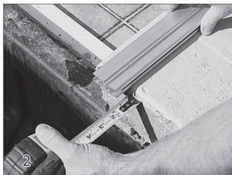
Cut the track (13) so it will extend from the front edge of the coping at the far end of the pool to 1" past the inside of the cover box if no encapsulation is being used. When encapsulation is used, it will extend one inch past the inside of the cover box, with the track extending one inch past the end of the encapsulation.
