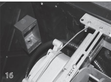
Attach the #8 copper bond wire (36) that is stubbed into the cover box to the bonding lug on the motor end of the mechanism.
