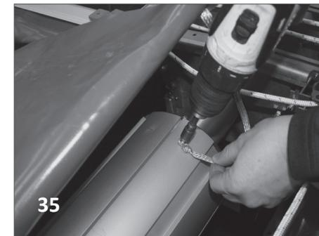
Using a self-tapping screw (30), attach the bonding wire on both sides of the roll-up tube.
