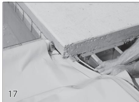
Continue to pull that one side of the cover into the track so the leading edge loop is over the water of the pool.
