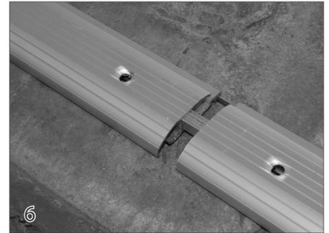
Join the track sections together by hand.
