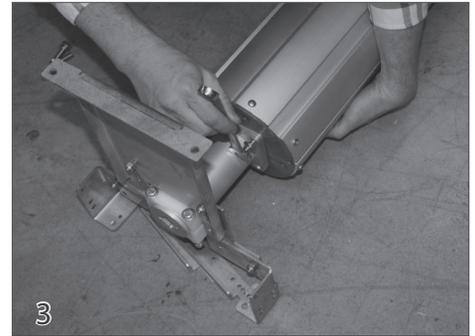
Attach the roll-up tube to the non-motor end of the mechanism using the 3/8" x 1-1/4" bolts (44) and lock washers (50) provided.
