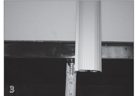
Cut the length of the track on each side of the pool so it will extend 1 inch past the inside edge of the cover box at the mechanism end.
