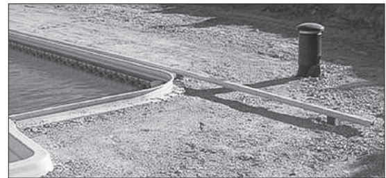
(4.a.) Track staked in place, ready for pour
