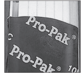
(3) Track protected by 2" 10 mil plumbers tape
